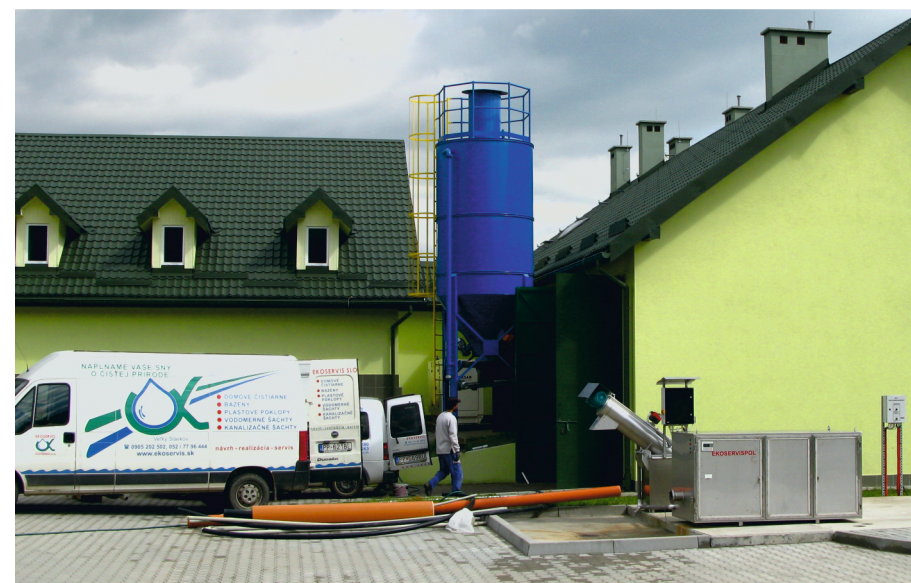
Automated sewage water intake station at WWTP building
