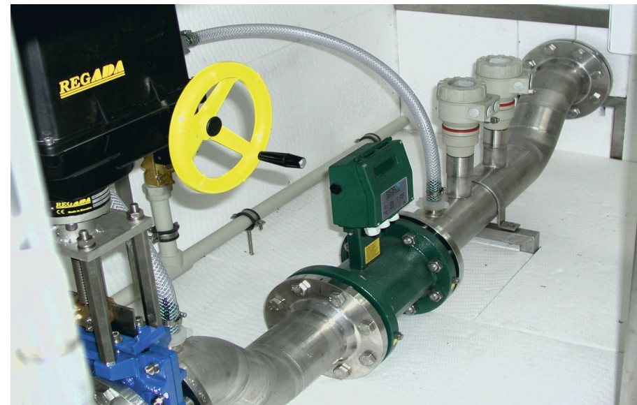
Automatic sewage water intake station with coarse pretreatment
